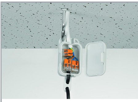
Pendant light connection in a suspended ceiling
